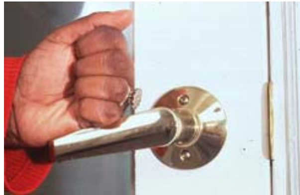
Example of a Universal Design Door Handle Photo from the Center for Universal Design Website
